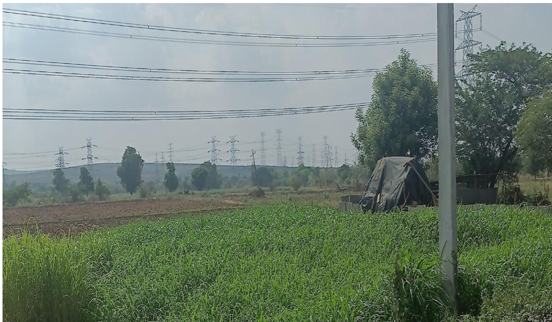
FIGURE 6-2 : EXISTING LINES GOING THROUGH CORRIDOR OUTSIDE CHINNAKAMPALLE SUBSTATION
